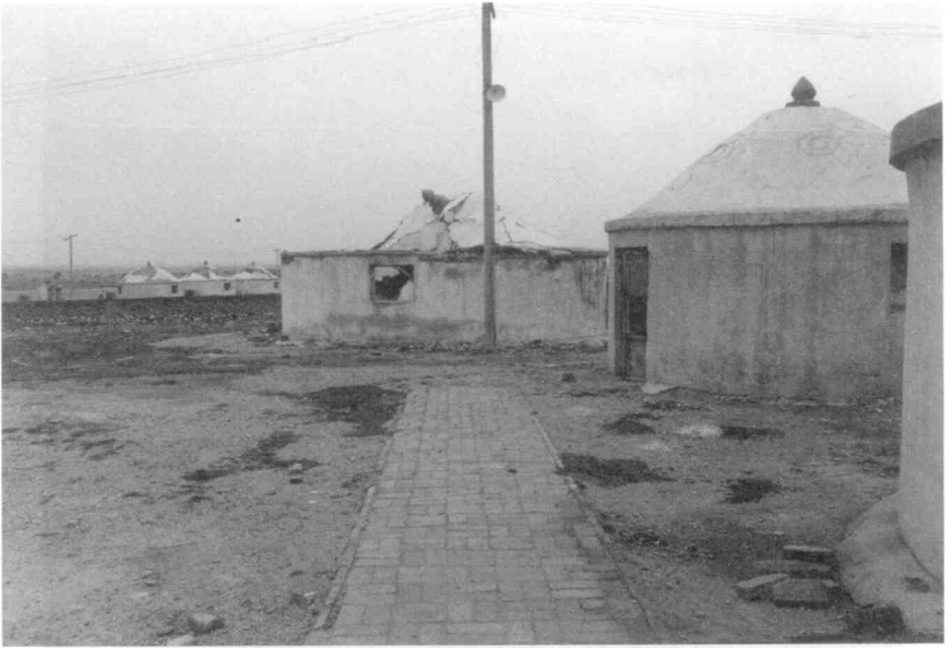
FIGURES 7-8 The Mergen Tourist Camp (east side). Above a shower/bathing 'yurt' with collapsed dome (Figure 7); note its more ornate boss when compared to the sleeping unit on its right and also below in Figure 8.
